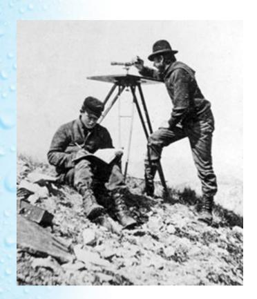
Surveyors would conduct topographic surveys by setting out a 50' or 100' grid, and using a Plane Table, determine elevations. Then, they would collect "Model Key Points", obvious low (or high) elevations, and breaklines, places where the elevation changes abruptly. The spot elevations and breaklines would be represented as a "contour surface"
